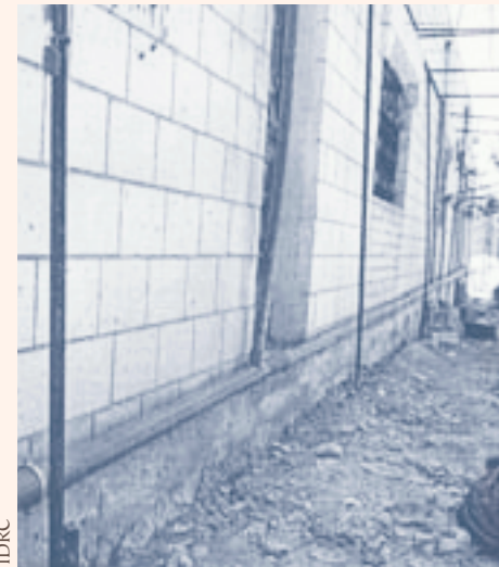
Grey water collected in piping along exterior walls of households
