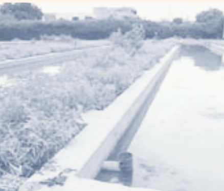
Saturation ponds where grey water from surrounding houses is treated
