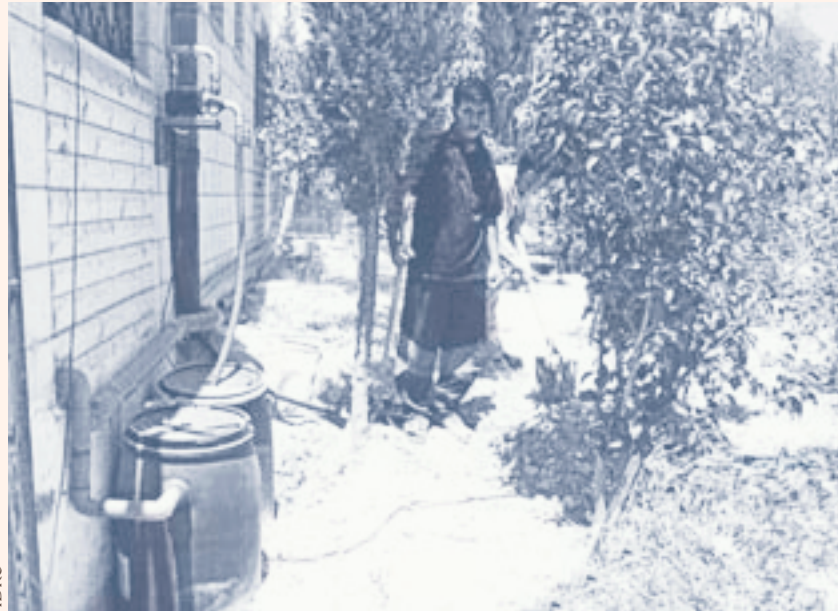
In Jordan, INWRDAM have trained a plumber who, in turn, is training others to install the systems
