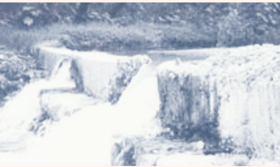
A diversion point in Guanajuato River for the irrigation canal
