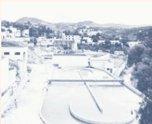
An overview of the Treatment Plant in Guanajuato, Mexico
