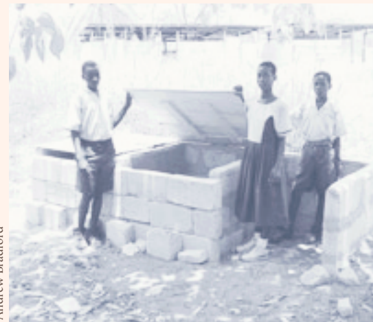
Block-built triple chamber compost bin being used at Apeadu Junior Secondary School, Kumasi
