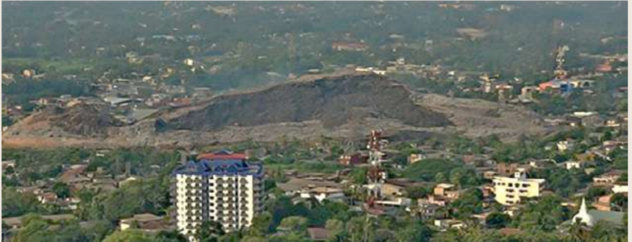
Meethotamulla dumpsite collapse (dark area shows where the landslide went down) (Source: ©SLAF media)
