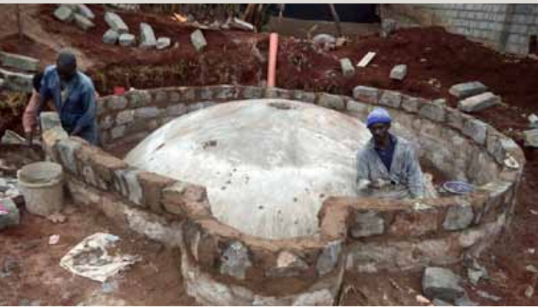
A biocentre under construction source: Practical Action
