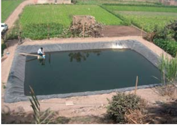
Stabilisation ponds reduce contamination risks Photo: IPES
